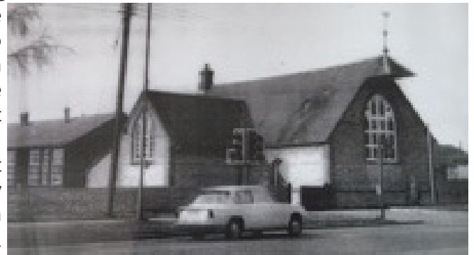
Crockwell School with wooden hut extension - 1970s
