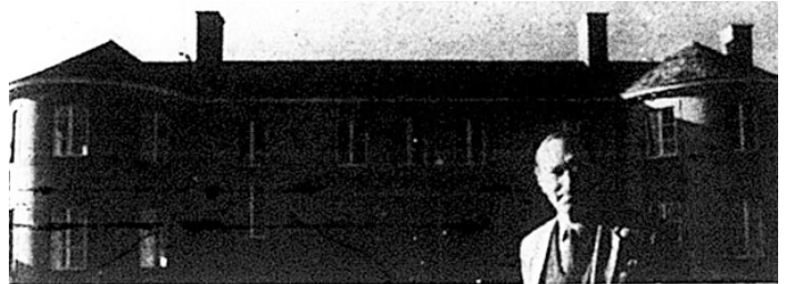
Col. Anson in front of Tusmore Park House, which the owner wants to demolish
